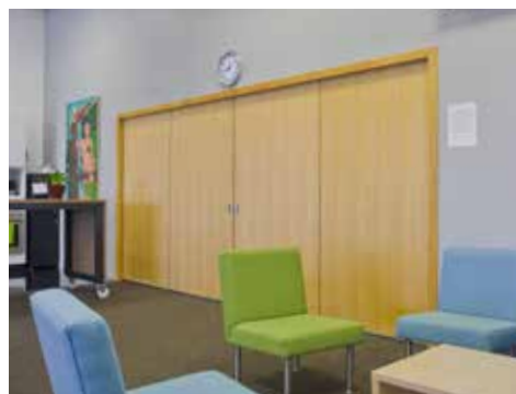
Bi-Parting acoustic doors (STC 35 / RW 35 dB)
